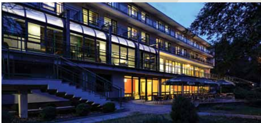
GREEN PARK CONFERENCE CENTRE – KAMPUS IBD BUSINESS SCHOOL W SEROCKU
